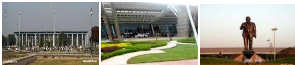
Figure 9: Images showing Nagpur international airport
